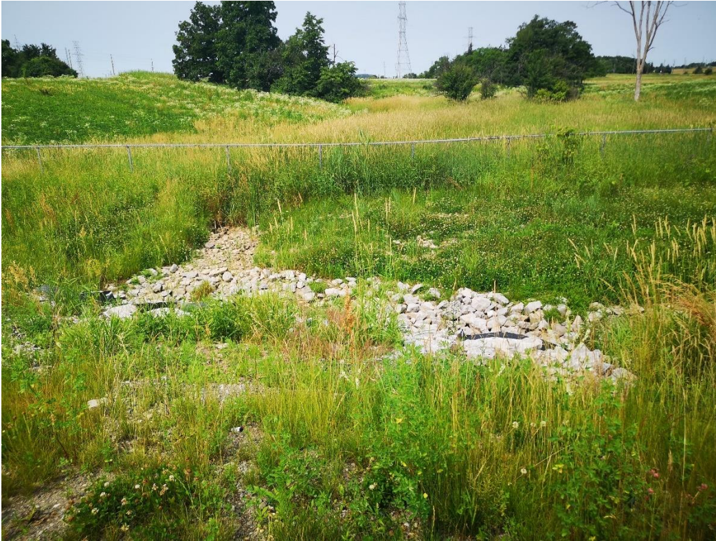
Upstream end looking west
