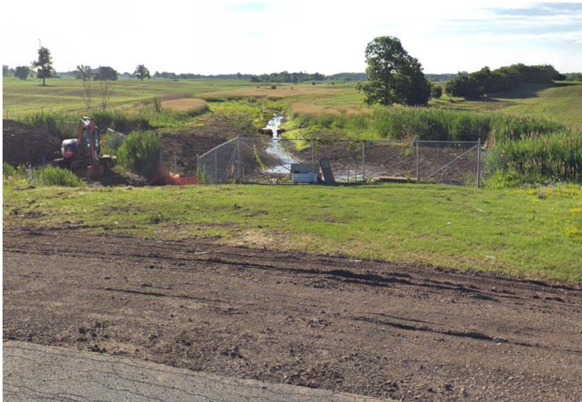
Downstream end looking east
