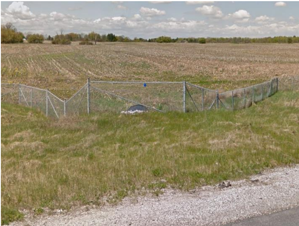
Upstream end looking west
