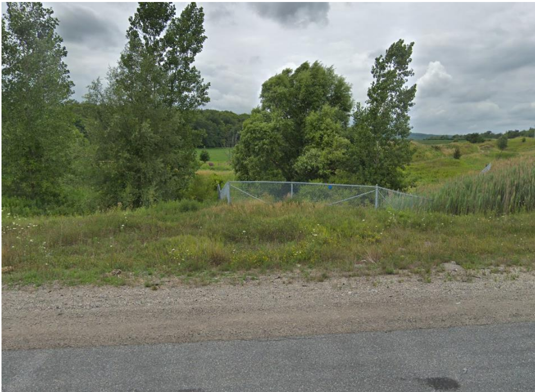
Upstream end looking west
