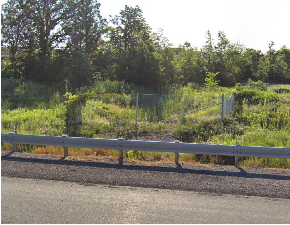
Downstream end looking east
