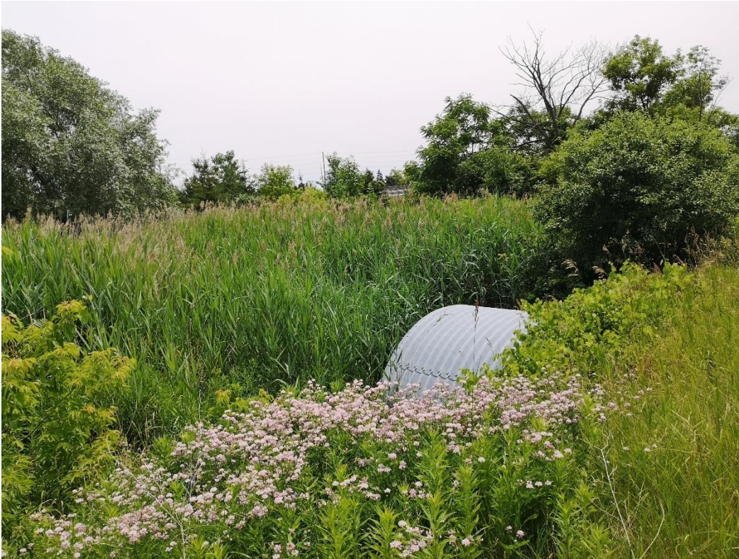
Downstream end looking east
