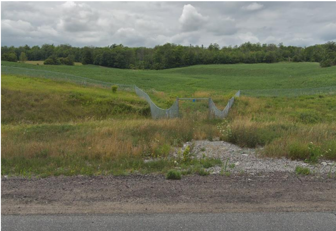
Upstream end looking west
