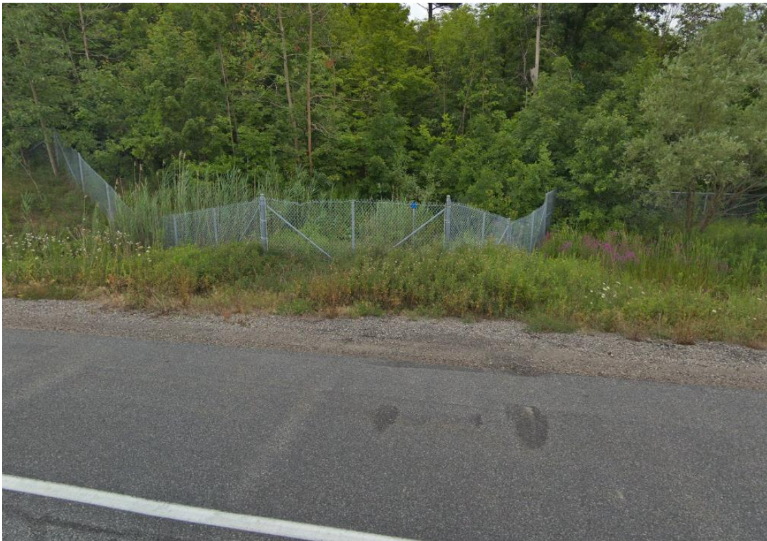
Upstream end looking west
