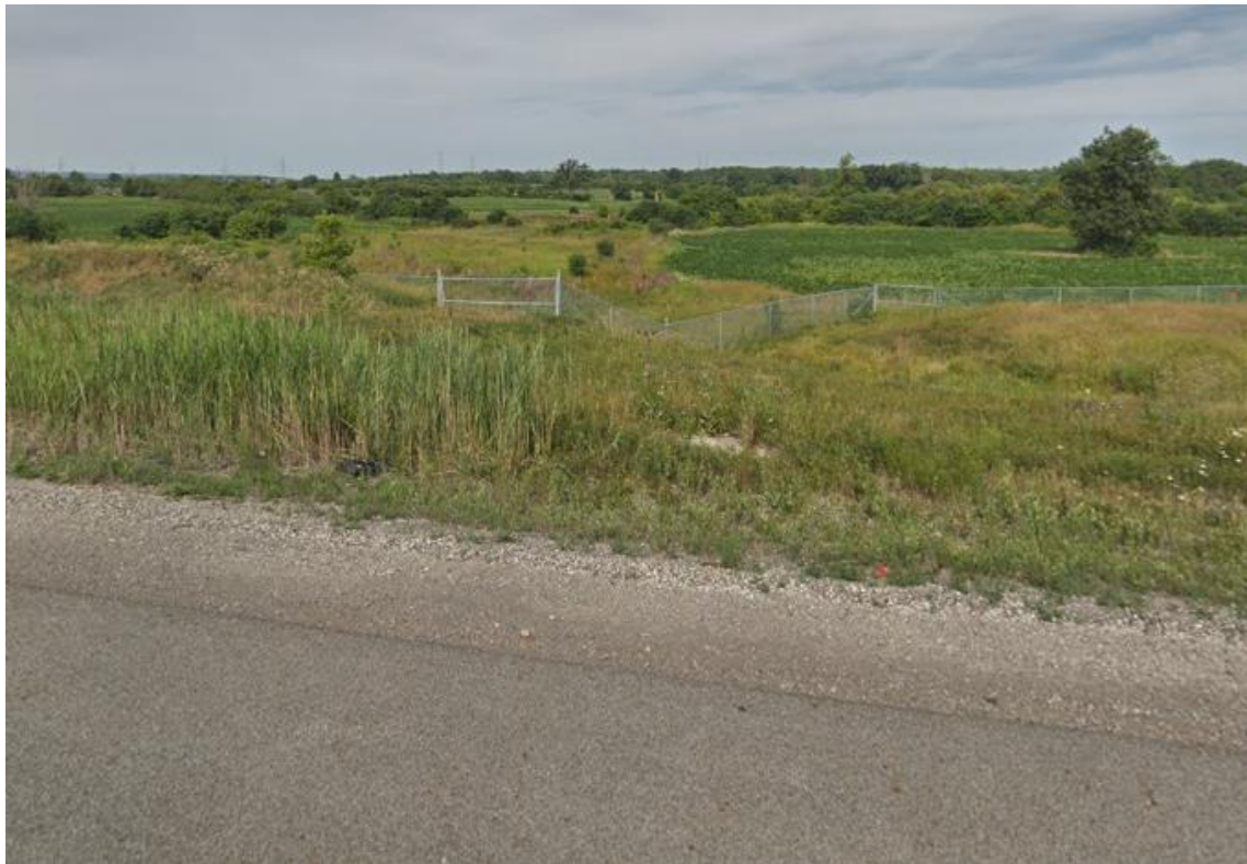
Upstream end looking west
