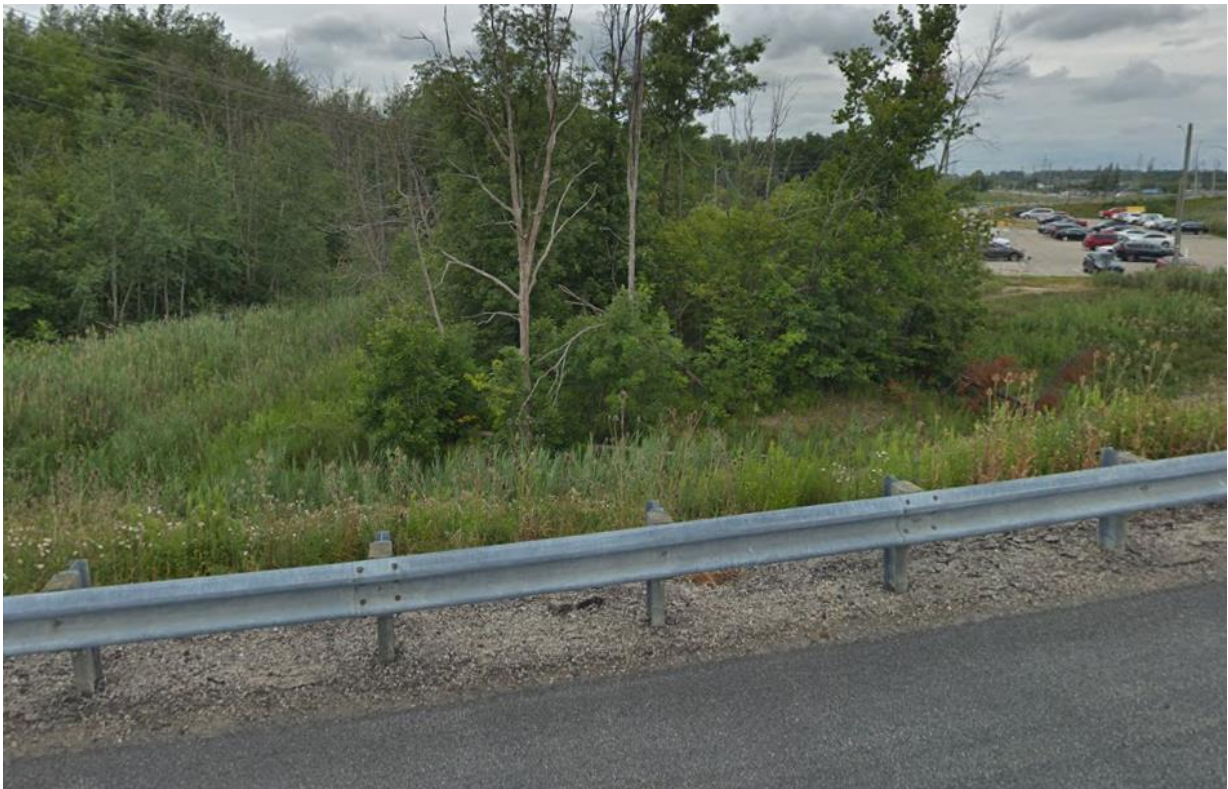
Upstream end looking west
