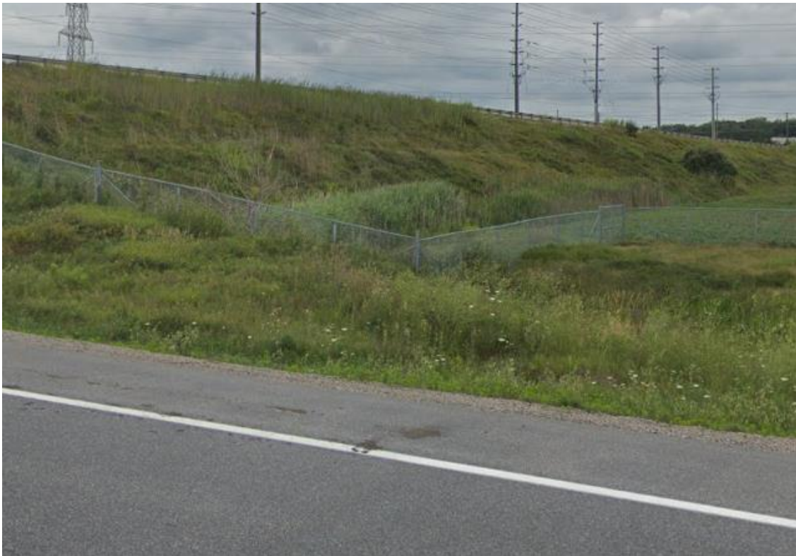
Upstream end looking west
