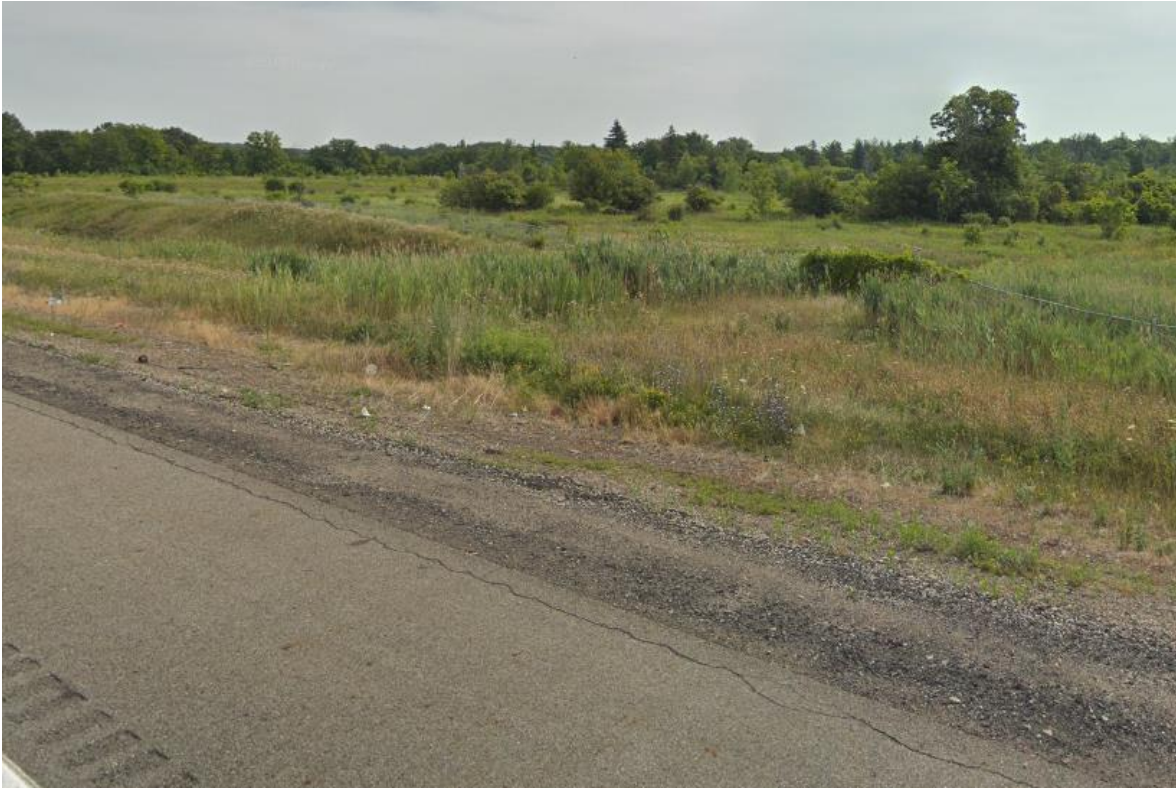
Downstream end looking east
