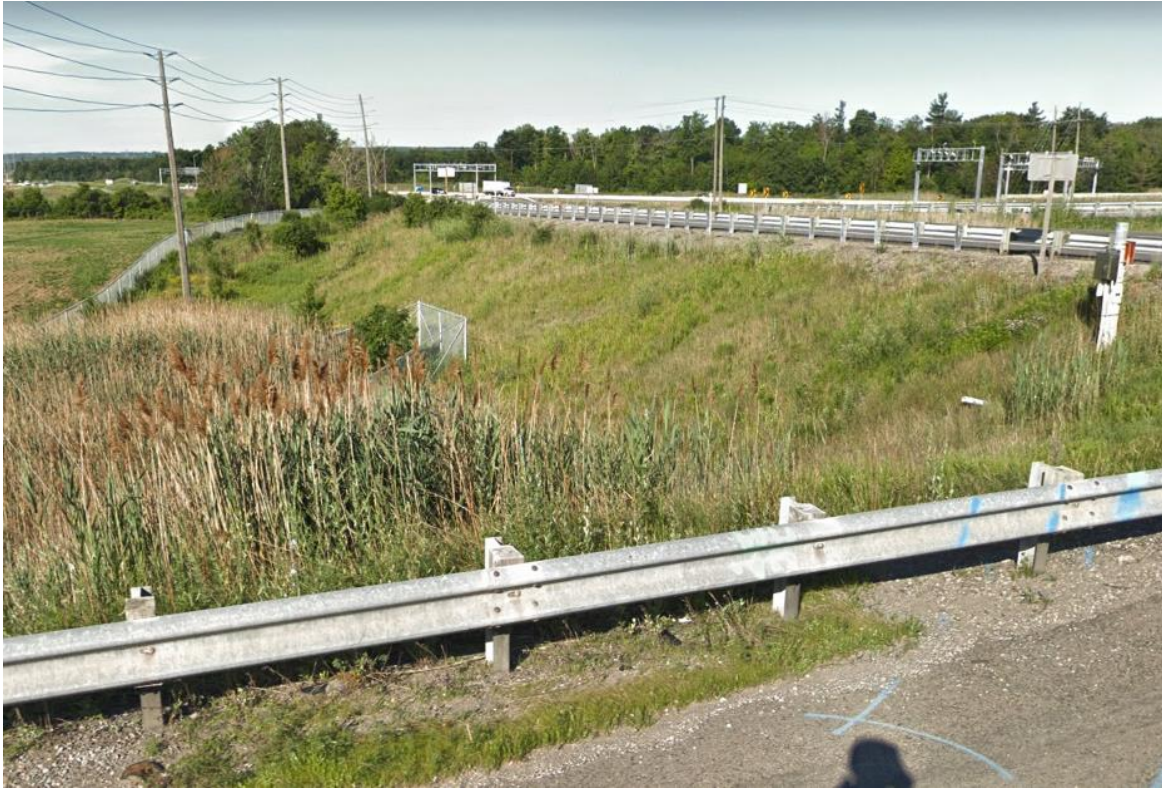
Downstream end looking south
