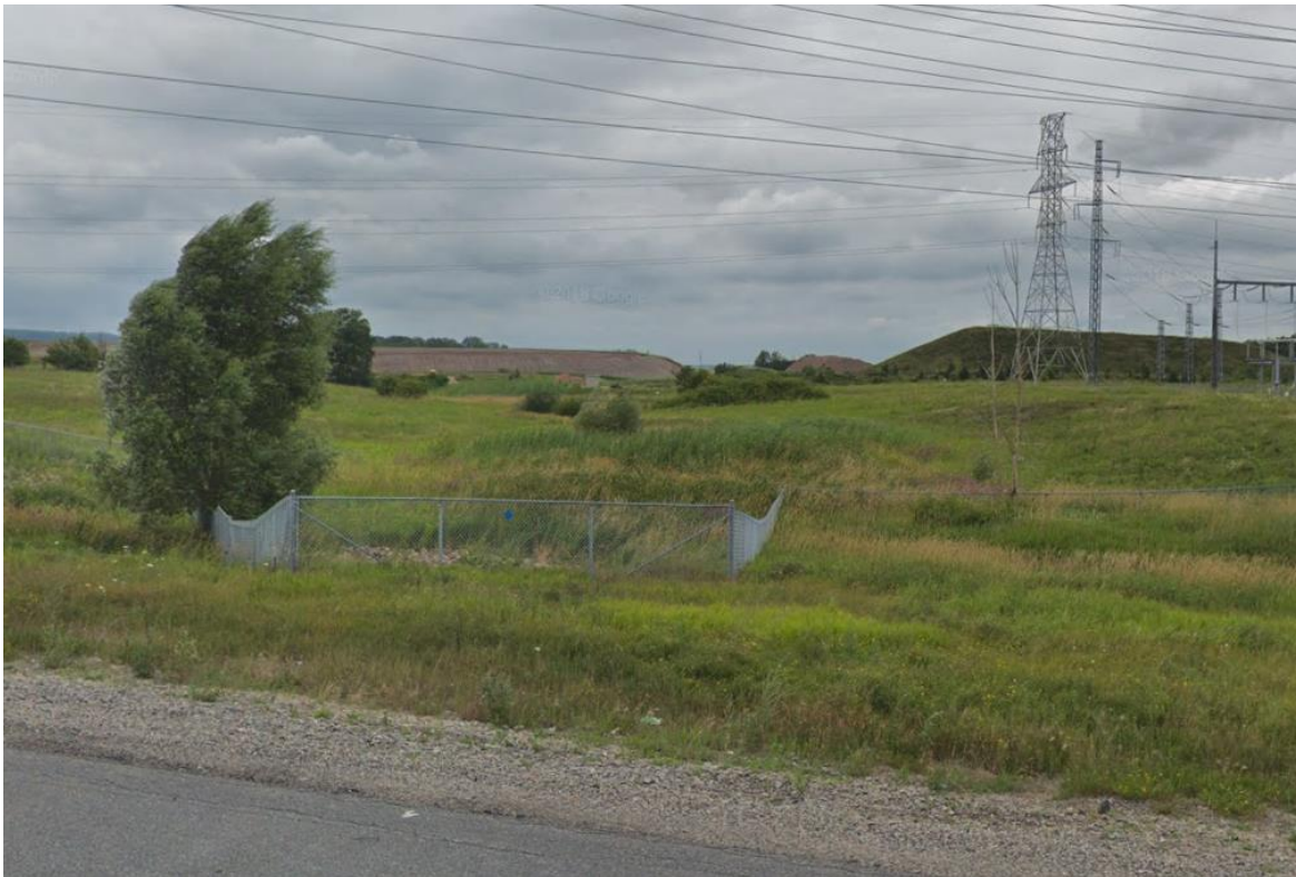
Upstream end looking west
