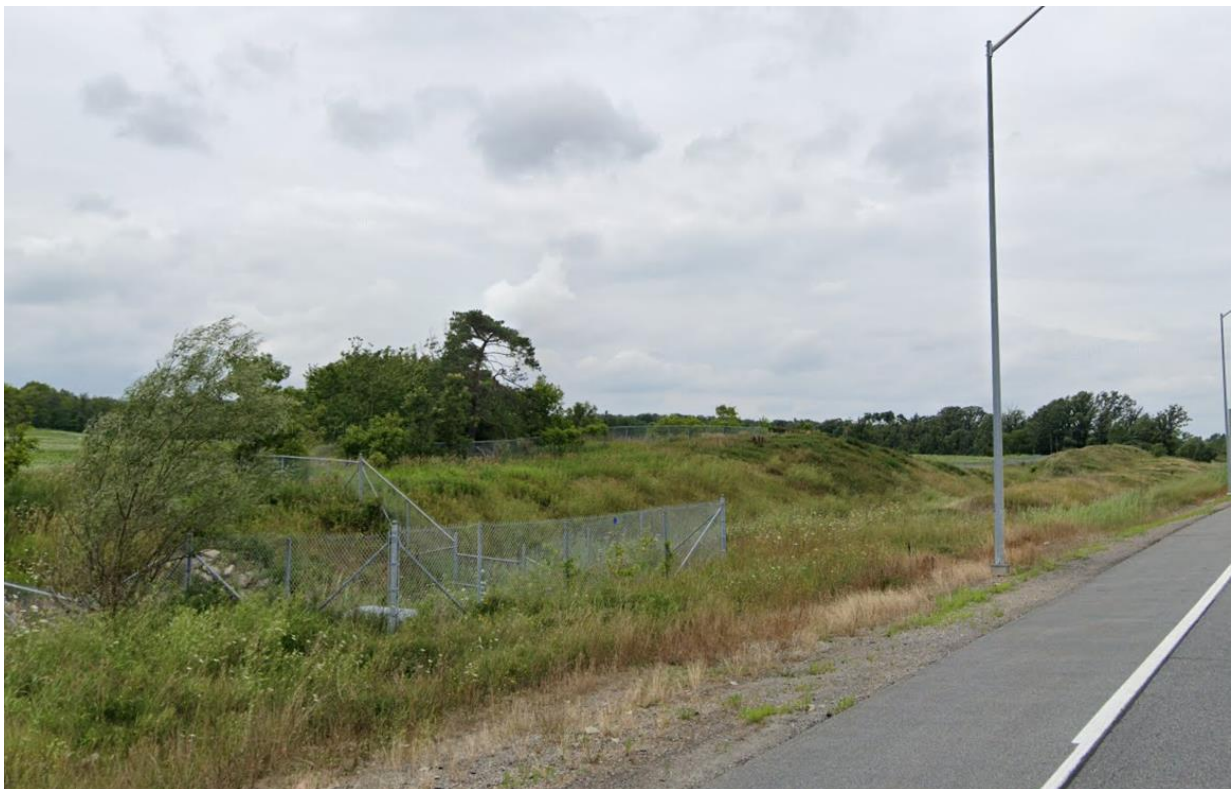
Upstream end looking north
