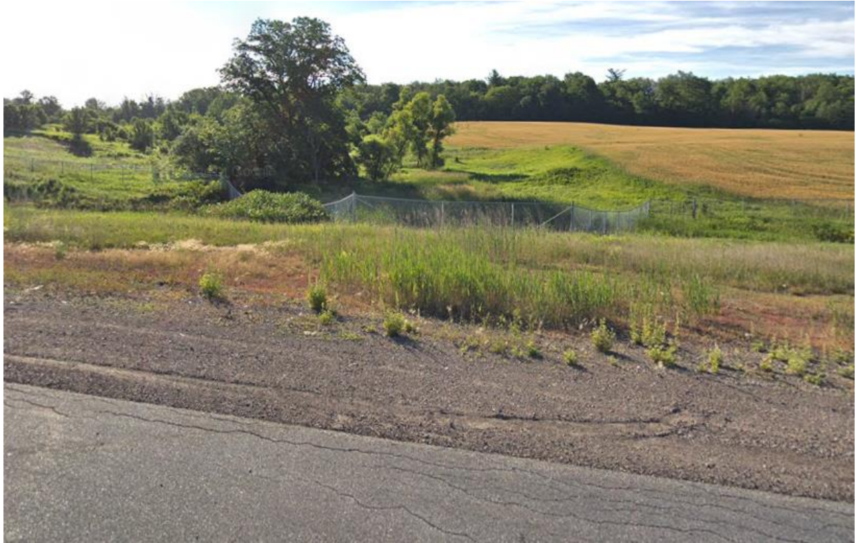
Downstream end looking east
