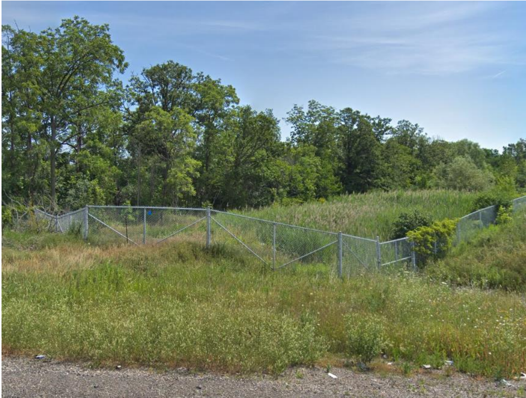
Downstream end looking east
