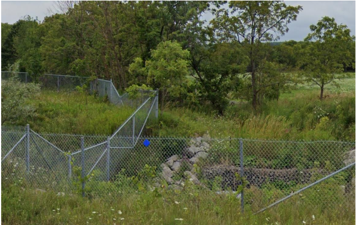
Upstream end looking west
